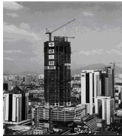
Fig. 7: SEG Plaza under construction
